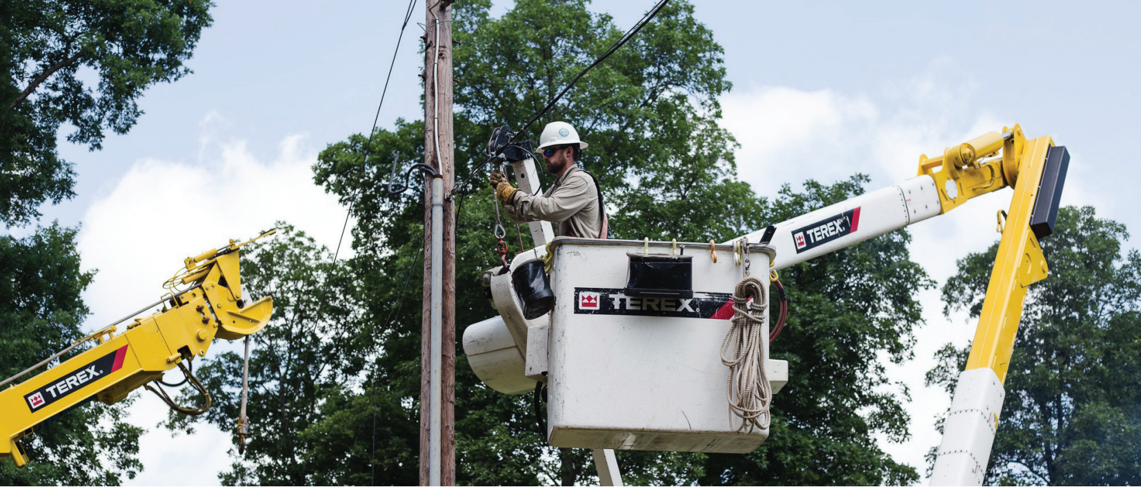
Apprentice Lineworker Landon Spencer prepares to replace a pole.
